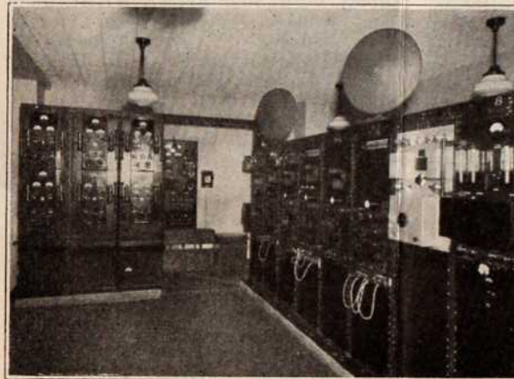
The Main Control Room of the Columbia Broadcasting System.
